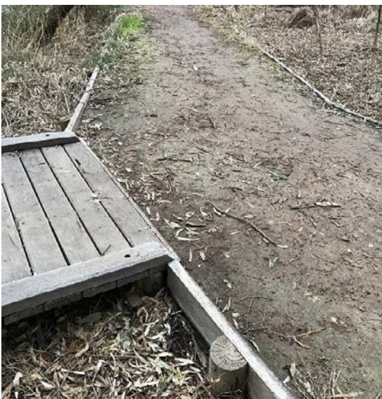
Image 10: Abutment edge connecting to the approach path
