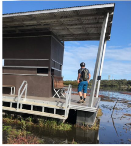
Bird hide with covered deck surrounds on pontoons allowing hide to move with the changing water level
