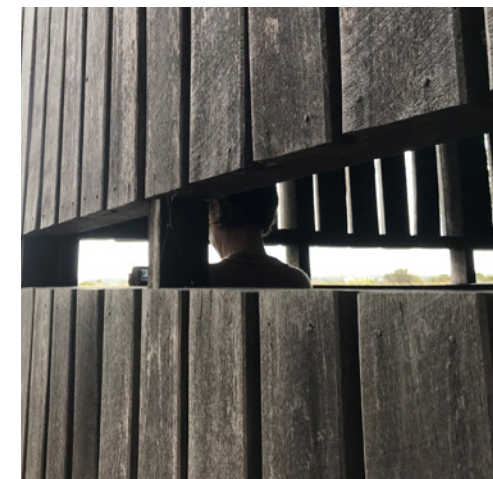
Timber battens with spacings to allow air circulation
