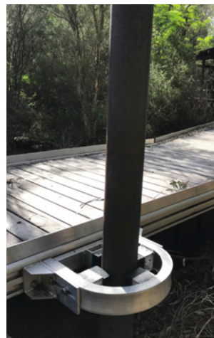
Structural piers for stabilisation at key locations along boardwalk
