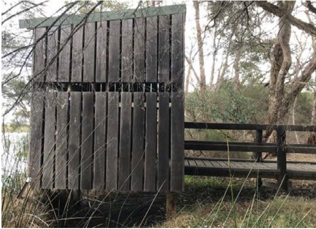
Image 12: Provide handrails along bird hide entry to contain access and for safety
