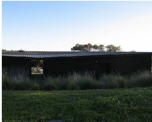
Horizontal timber clad structure that visually recedes into the wetland environment
