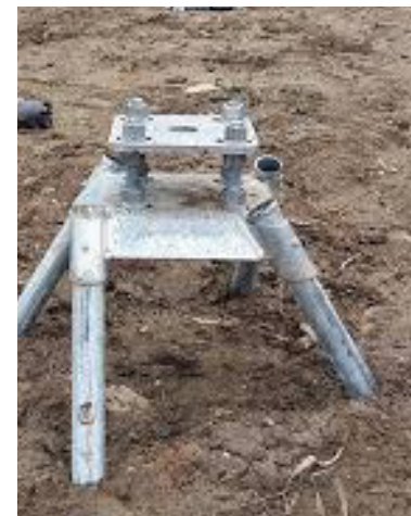
Concrete-less pile footings to minimise ground disturbance
