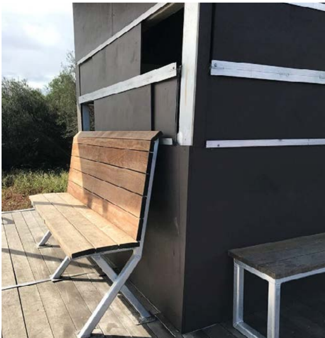
Image 18: External furniture that allows views from the interior increasing the functionality of the hide and structure
