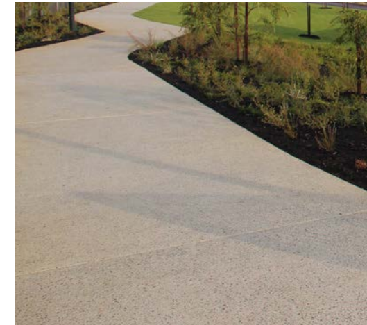
Coloured concrete paving to be used for the Arrival node and access path to bird hide boardwalk
