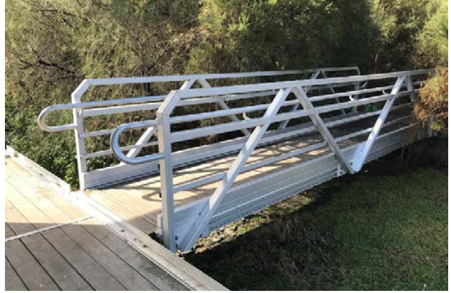
Image 2: Narma Kullarck Bird Hide gangway access with hand rails
