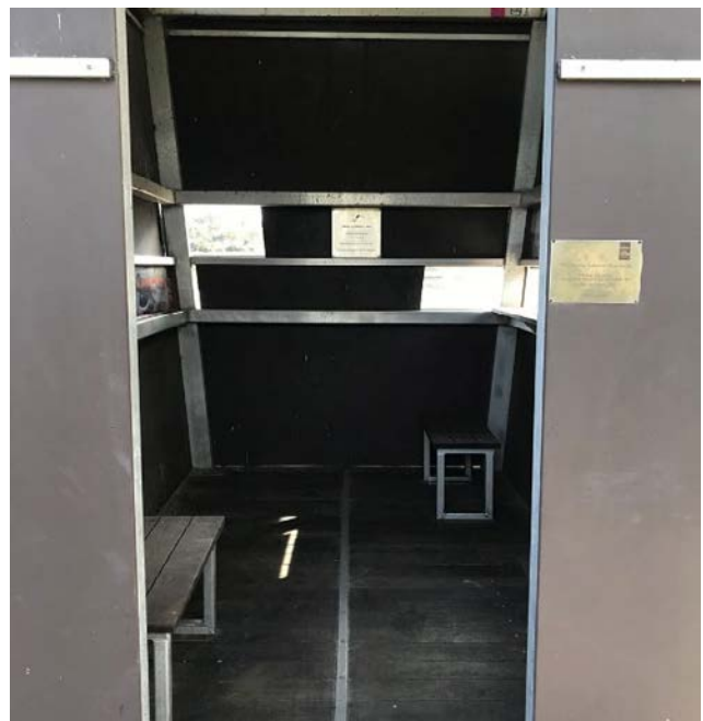
Image 19: Interior of the hide with window at varying heights to allow for a range of users
